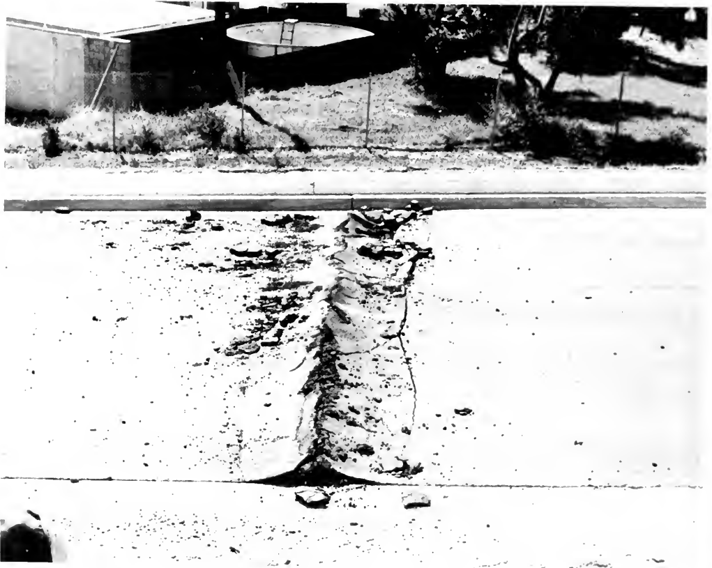
Photo 11. Compression buckle in asphaltic concrete ramp pavement on Route 210.
